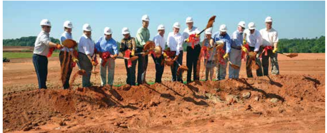
College officials joined Oconee County partners from government, education, and economic development to break ground on the Oconee Campus, the first building to be constructed on the site of the future Oconee County Workforce Development Center.
